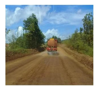
Dust is the prevalent problem in Nickel Laterite Mining. Laterite materials are so fine they become airborne during hot weather and turns into mud during rainy season.
